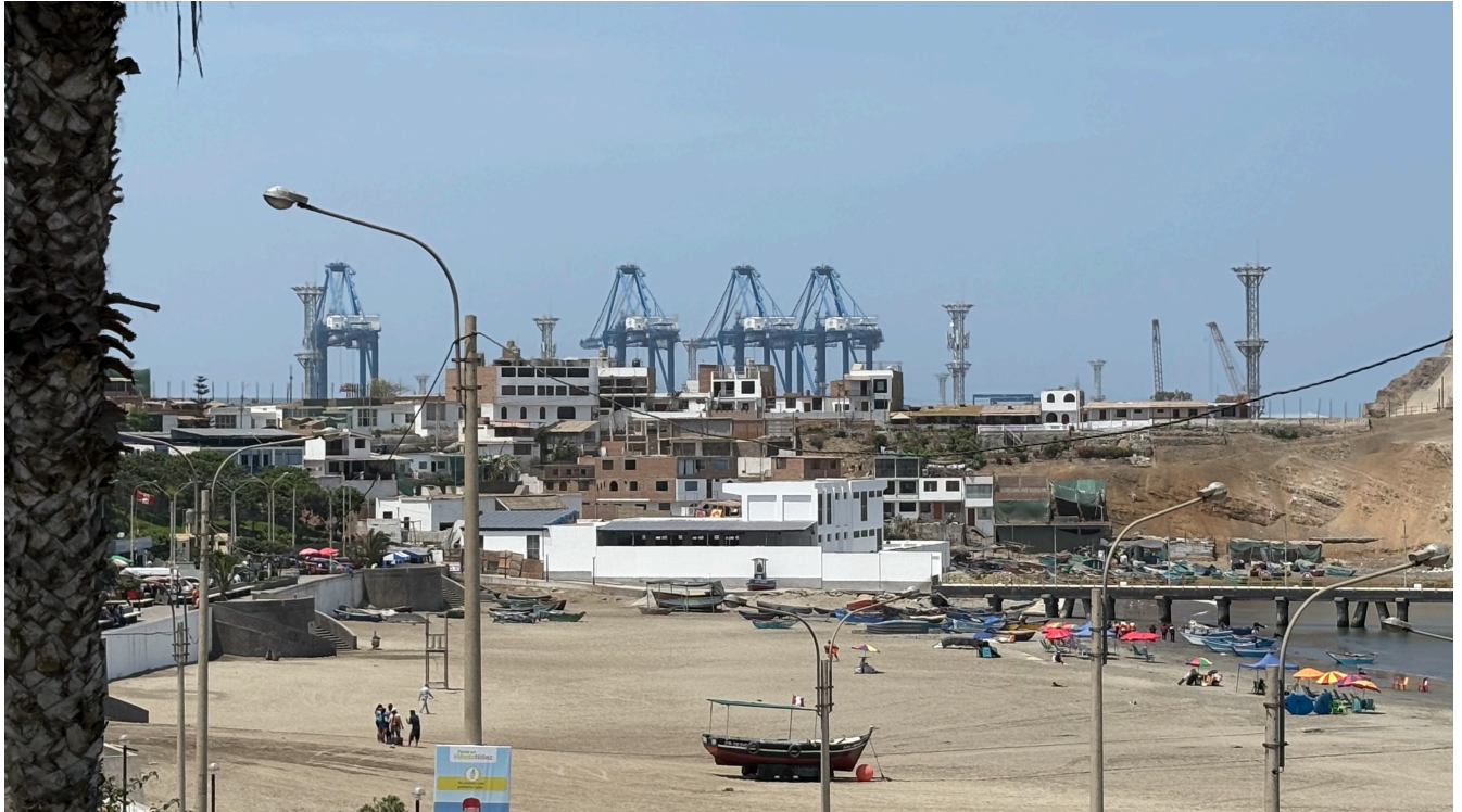
Figure 8: The juxtaposition of the traditional fishing activity being overtaken by the COSCO port in Chancay (IBI Consultants, November 2024)
